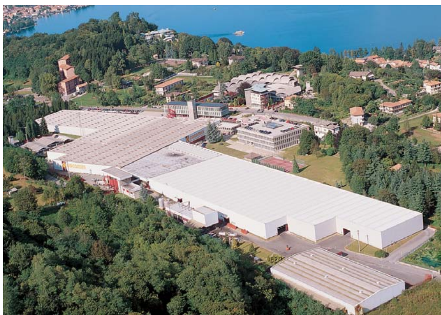
Main manufacturing facility in Italy
